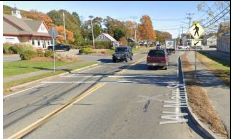
6 Example of crosswalk missing curb ramps
