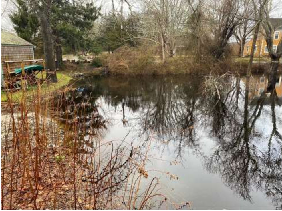
Marsh Side Culvert Outlet During Flood Event
