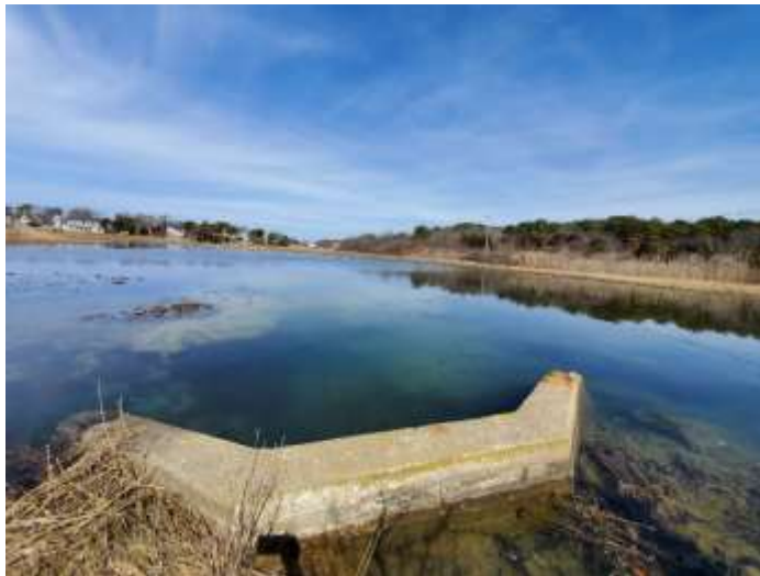
Culvert headwall and up-gradient salt marsh (taken 3-15-22).
