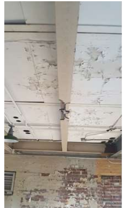
Photo 5: Steel Support Beam
