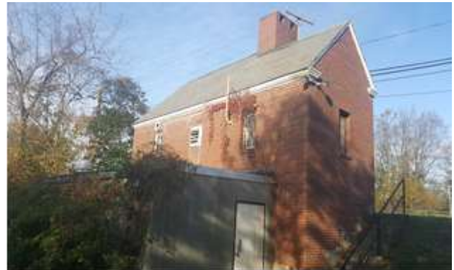
Photo 2: 91 South Street Rear
