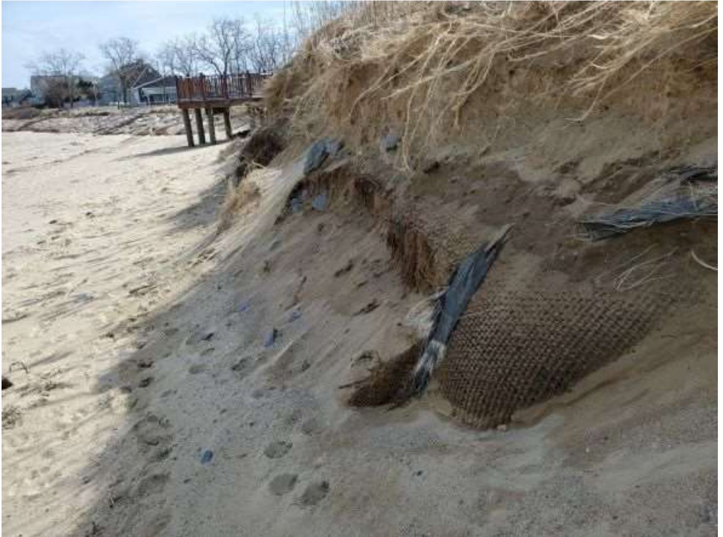
Storm Damage to Coir Roll System after Winter Storm Keenan (Picture taken March 2022)
