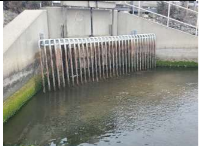
Tide gate near low tide – Photo taken April 2021
