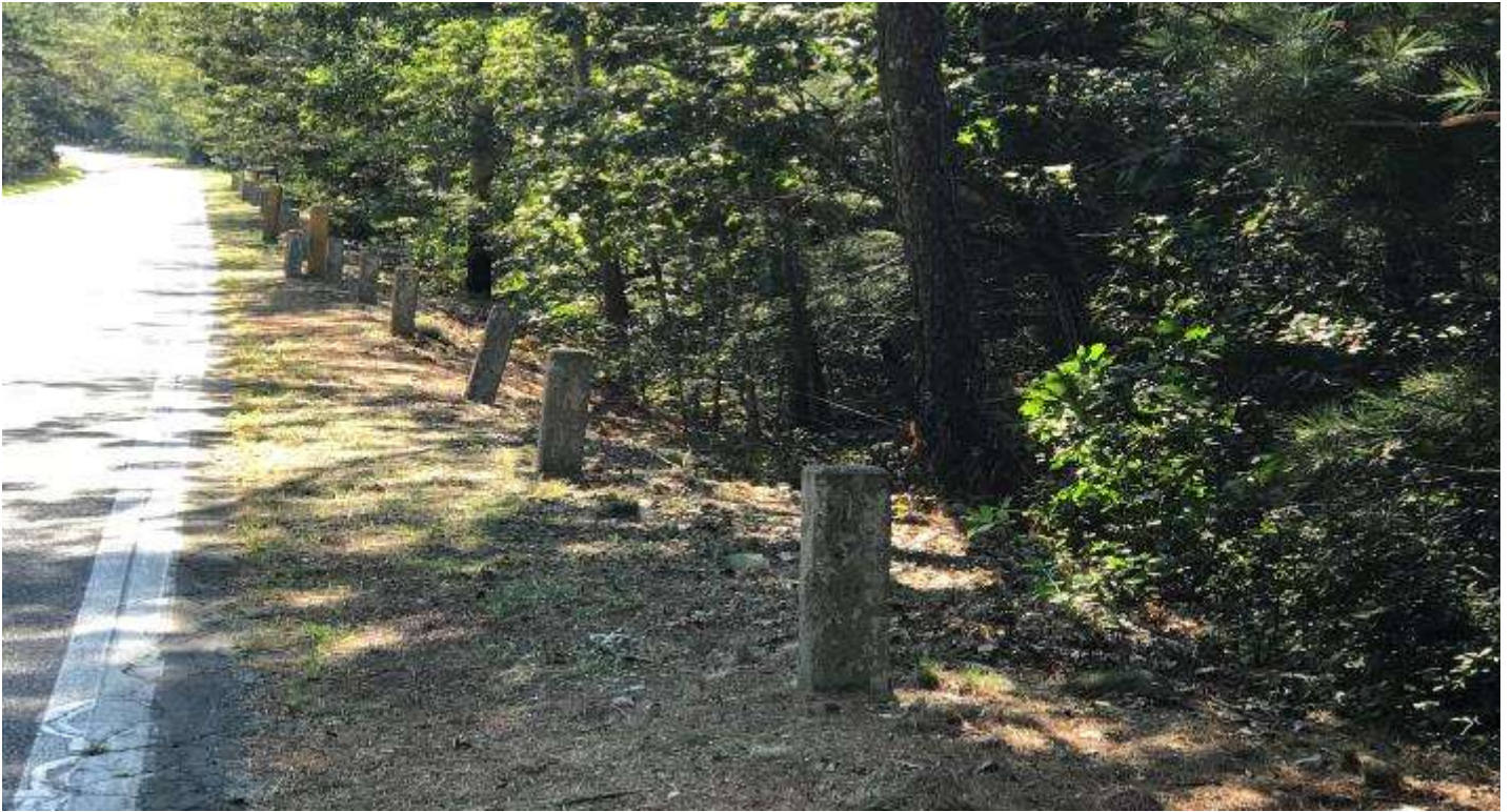
Concrete Guardrail Removal
