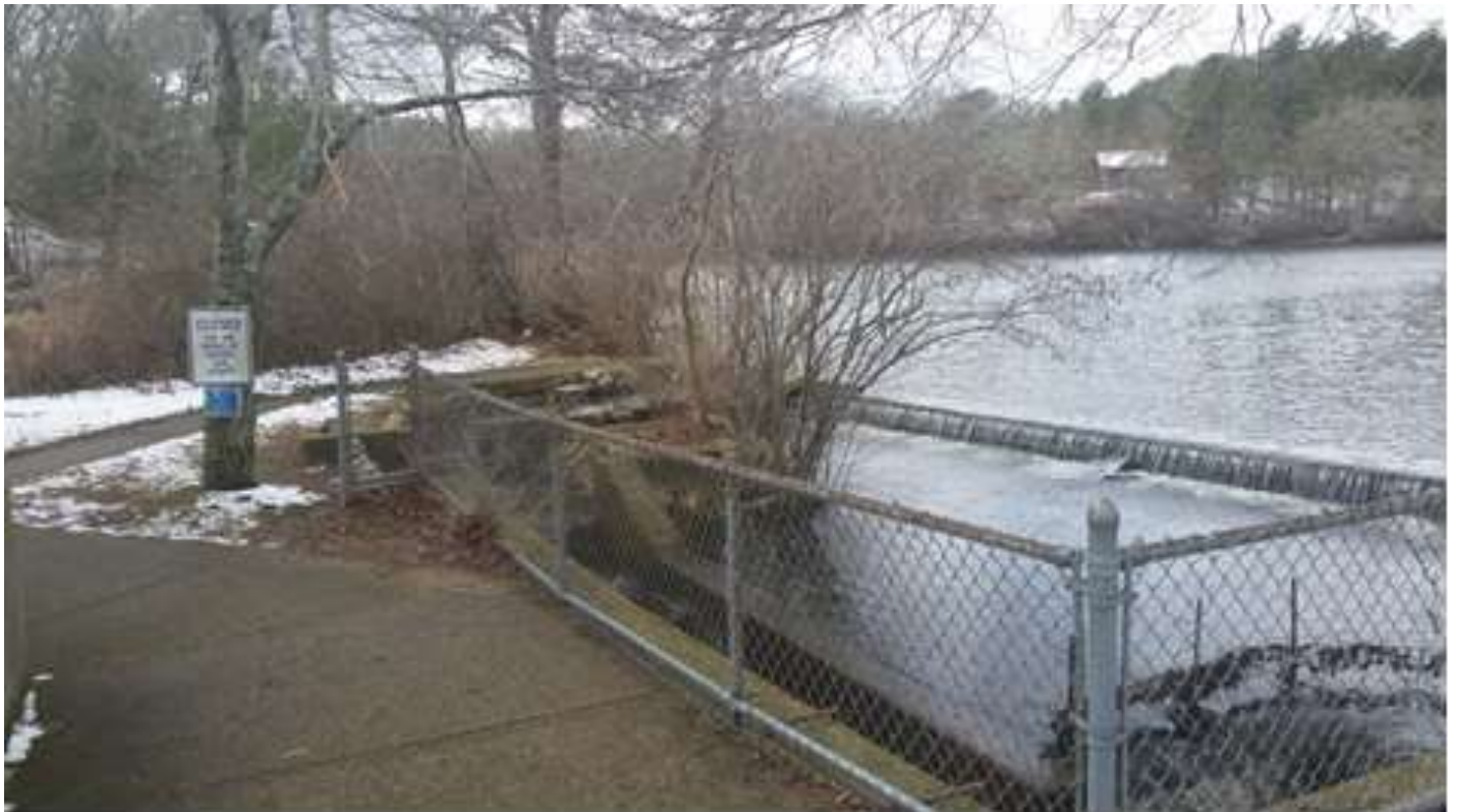
Mill Pond Dam and Fish Ladder
