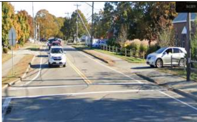
7 Low-visibility crosswalk and missing sign
