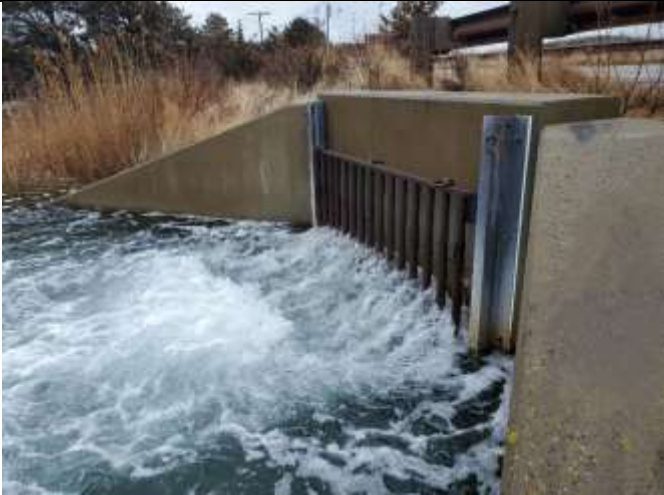
Upstream trash rack near high tide – Photo taken March 2023
